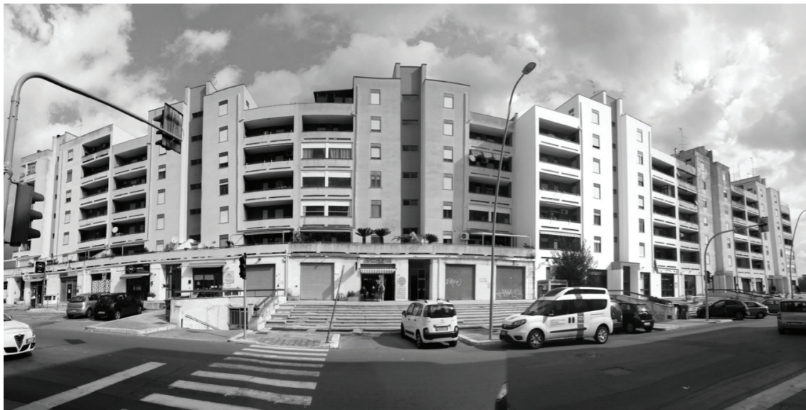
Fig. 6: Houses block in Via Taranto (photo by the author)
